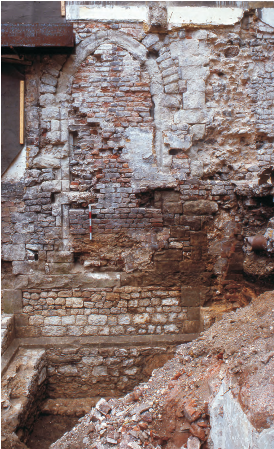
Fig 11 Black Friars: exterior view of one of the bricked-up windows on the north wall of the provincial prior's building (0.5m scale) (LAARC, site FRI88, image 975-89)
