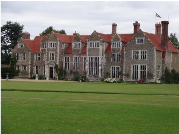
The north front of Loseley House. The house was re-roofed in 2015. Photograph by the author.
