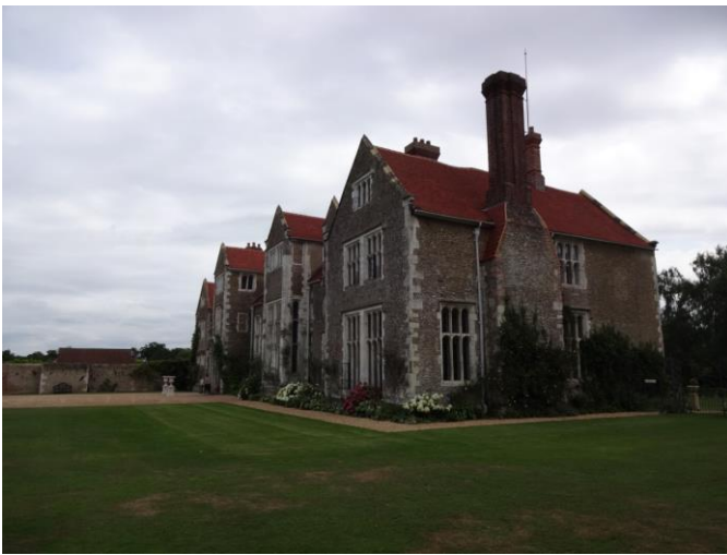
A view of Loseley showing the west wall of the house, which is where George More's wing joined onto the Elizabethan building. A patch of the stonework to the far right is paler than the rest, which may indicate work done after the wing was demolished. There is also some different coloured stonework to the left above the drawing room window. Photograph by the author.
