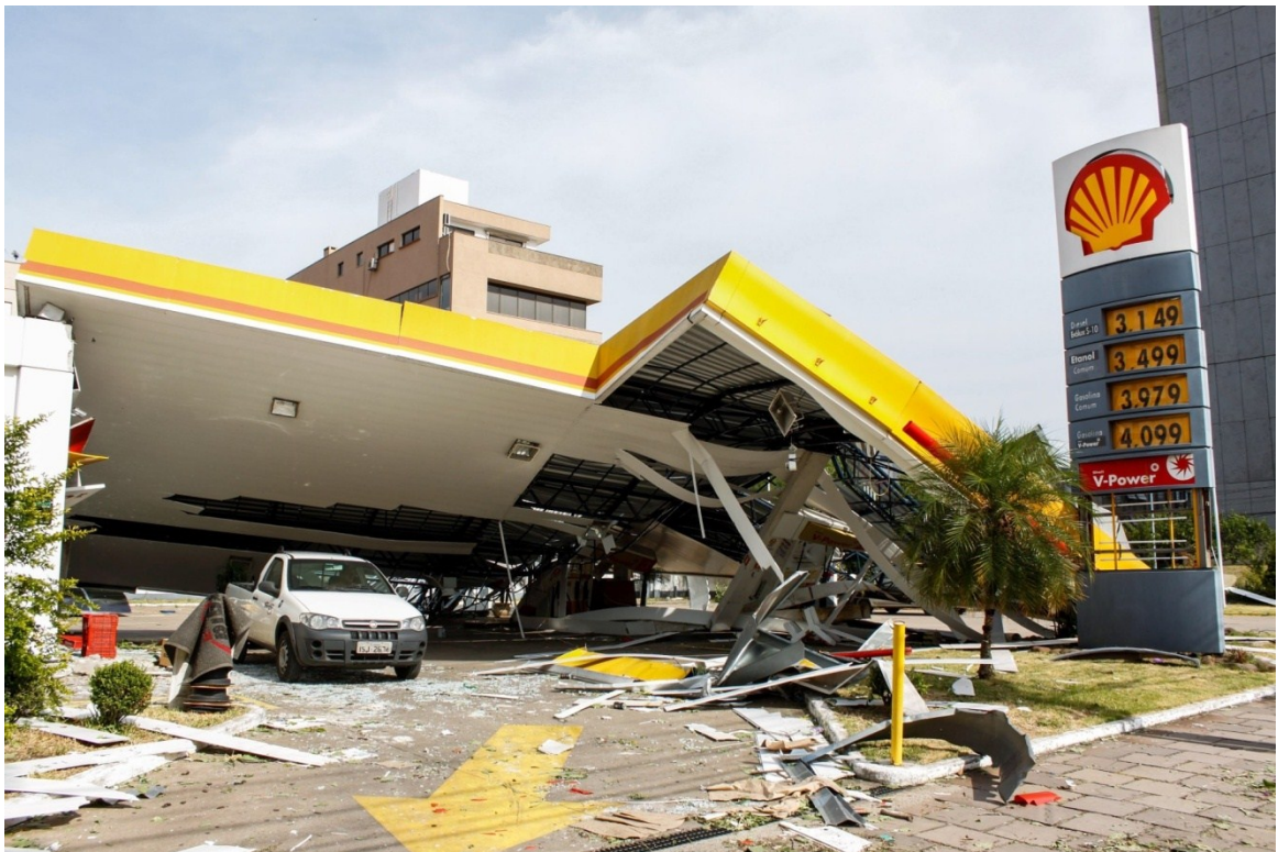
Figure 77: Destroyed gas station. (G1, 2016)
