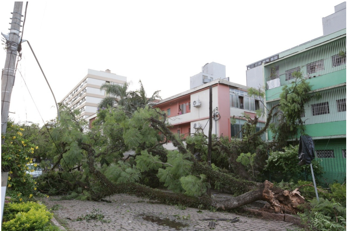
Figure 75: Fallen trees, squashed power lines. (G1, 2016)
