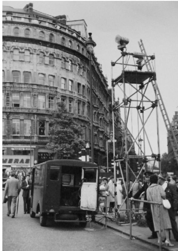
Figure 60: CCTV camera installed to monitor crowds and traffic during Thai royal family visit, July 1960 (EMI Electronics Ltd). 642
