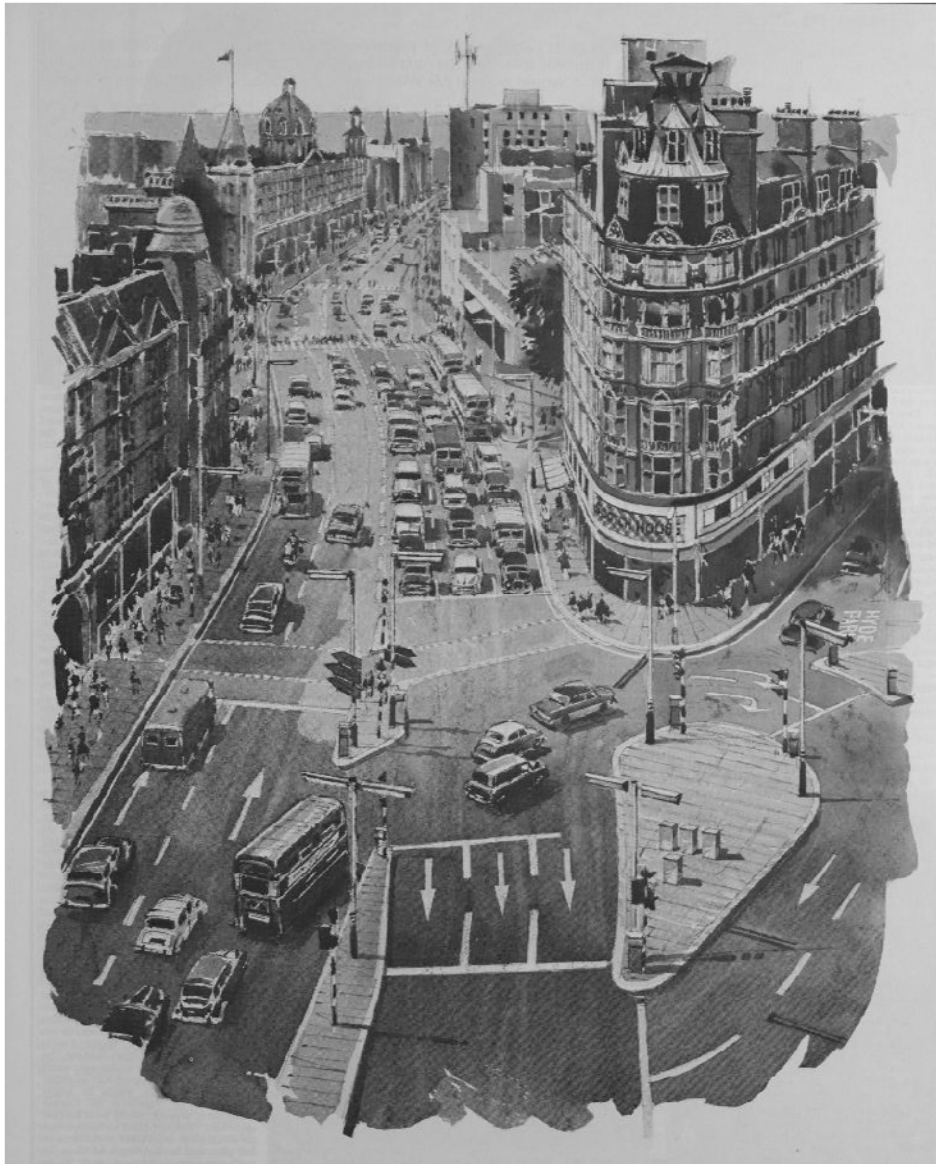
Figure 53: Artist's impression of Knightsbridge junction, showing equipment boxes on right-hand traffic island, 1967 (© Illustrated London News Ltd). 581
