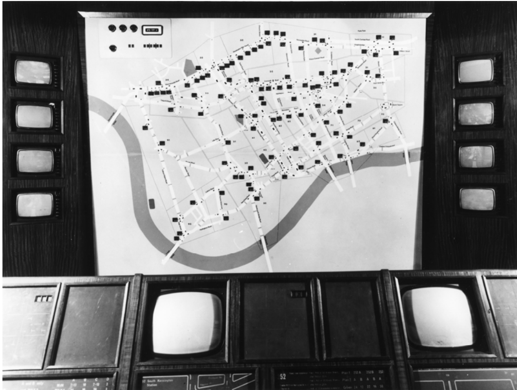
Figure 52: West London Traffic Experiment control room showing map and CCTV monitor screens (© Metropolitan Police Service, courtesy of the Metropolitan Police Heritage Centre). 580
