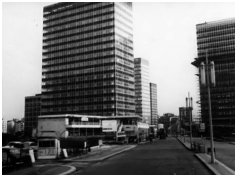
Figure 65: London Wall and its tower blocks, c.1964 (Courtesy of the BBC). 694
