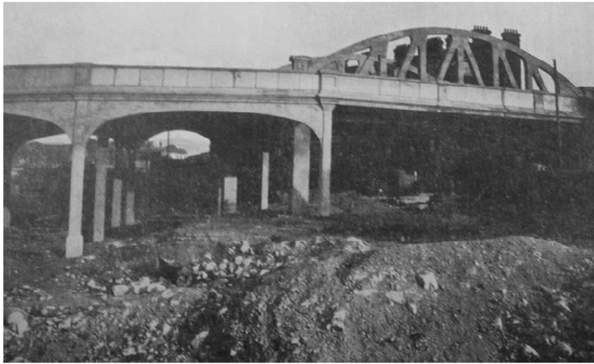
Figure 27: Part of Dover Borough Council congestion-relief viaduct and bridge system, completed 1922 (Concrete and Constructional Engineering). 279
