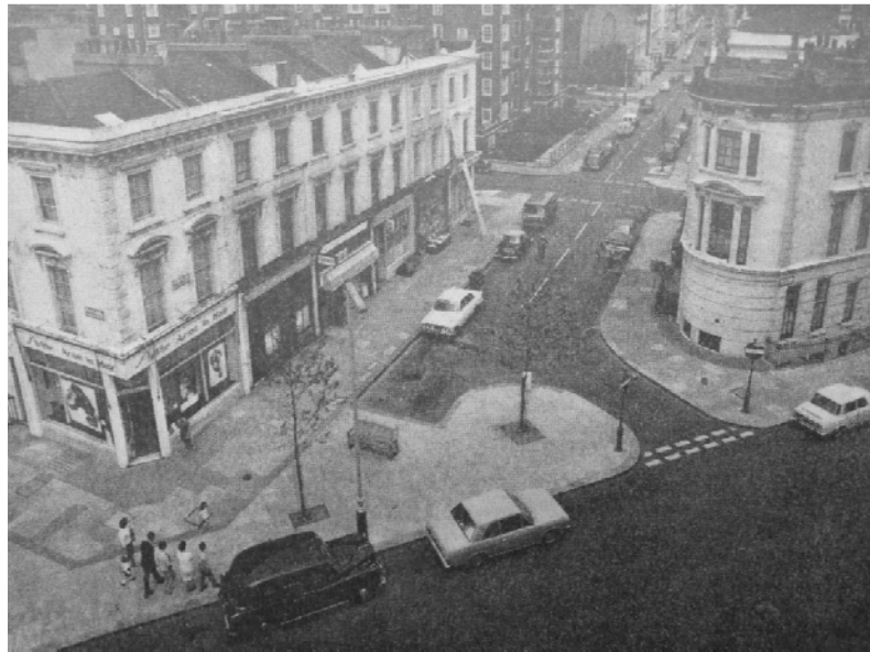
Figure 61: Exit from Charlwood Street into Lupus Street, Pimlico, showing footpath widening and conversion to one-way traffic with parking bays, c.1969 (Courtesy of Westminster City Archives). 659
