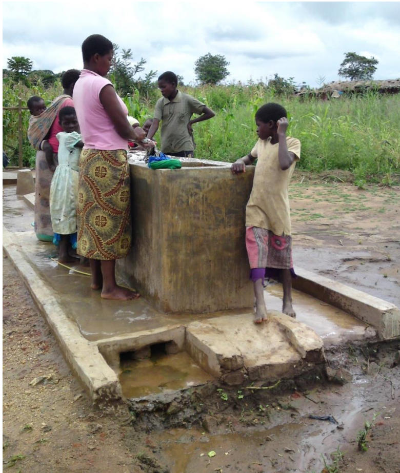
Plate 6.9: Drain Water from a Borehole Flowing into a Water-point Garden
