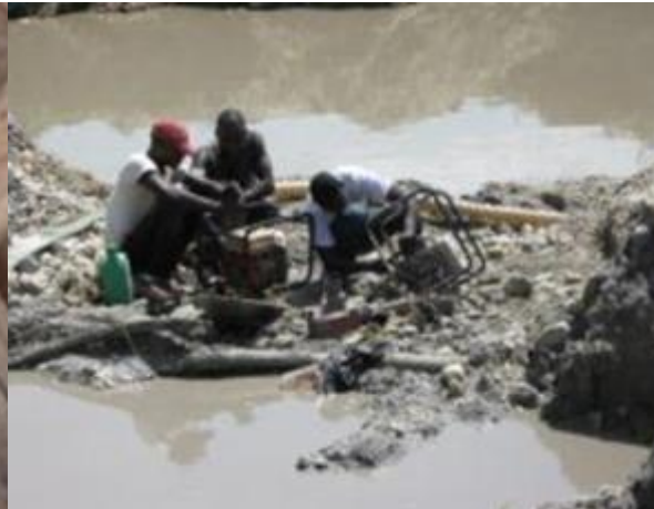
Technicians repairing a water pump in Mboscoro
