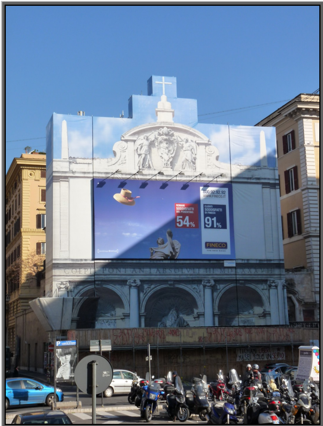
Figure 62 Wrapping on Moses Fountain during restoration (2009)
