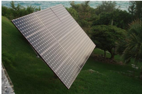
Plate 9: A ground-mounted bank of solar photovoltaic panels in the yard of a wealthy resident (Author 2011).
