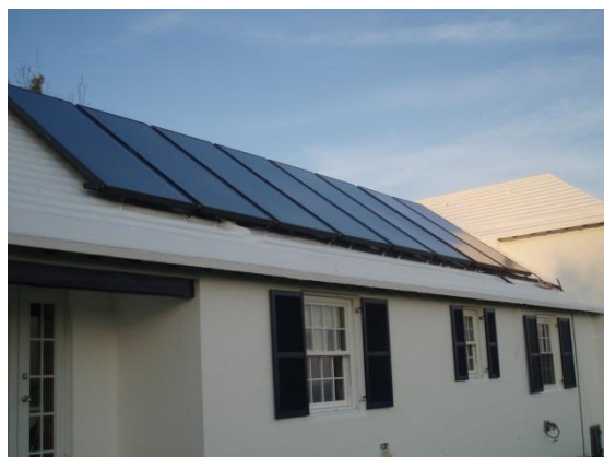
Plate 8: A bank of solar thermal panels on the roof of a wealthy resident (Author 2011).
