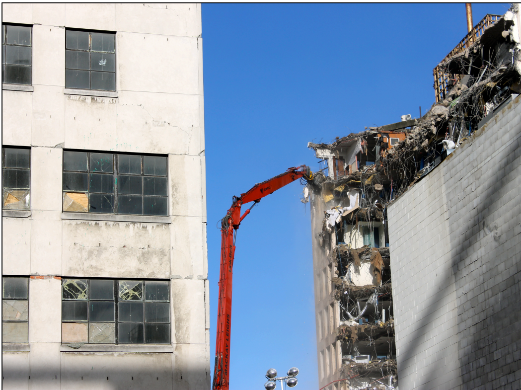
Figure 7.4 Demolition in Christchurch CBD (Stephanie Morrice 2012)
