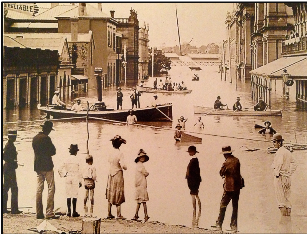
Figure 1.1 Creek Street, Brisbane. 1893 flood. (© Frozen in Time Gallery 2013)
