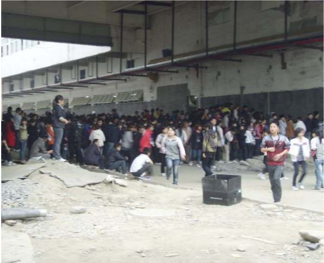
In a vast construction site of half-finished buildings, Foxconn Chengdu workers queue up to punch their time cards at 7 a.m. The polishing workers did not know that aluminium dust created by the polishing of an iPad could explode under certain conditions. Photo credit: Jenny Chan.
